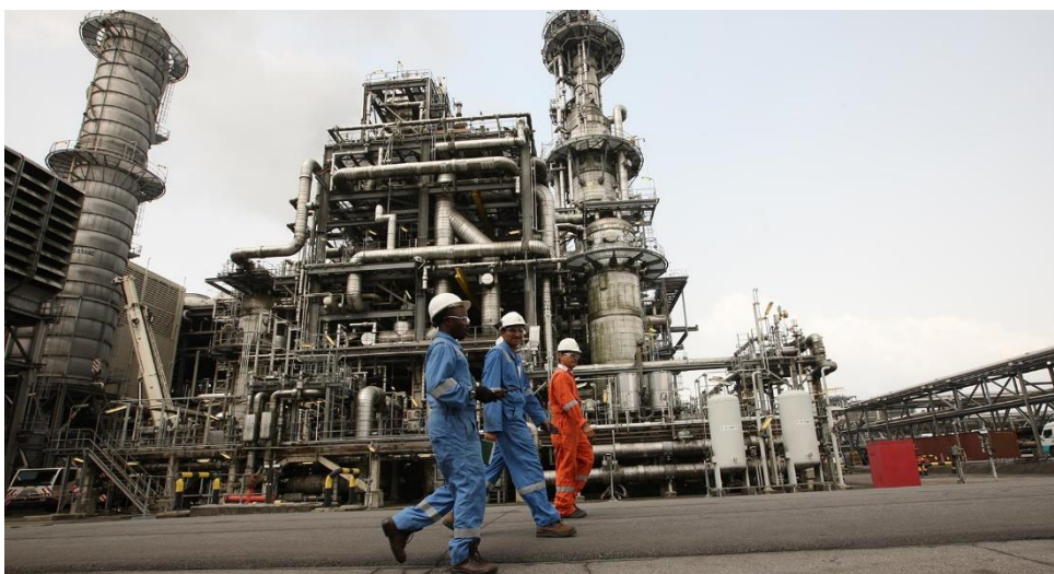
Nigerian Liquefied Natural Gas (NLNG) Facility in Bonny Island, Nigeria. A natural gas processing facility with production capacity of 22 million Tons Per Annum (Mtpa) of LNG and 5 Mtpa of Natural Gas Liquids from its six-train plant complex
