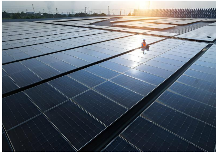
Set of Solar PVs being installed for renewable power generation
